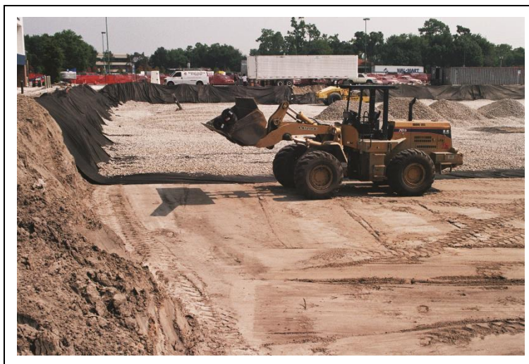
Figure 6 Installing foundation layer
